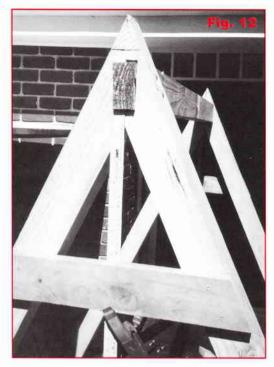
Cut the 65 degree angles on the workcentre in rip saw mode, using the protractor (**Fig. 13**). Drill and screw them to the frame sides with two 75 mm treated pine screws at each joint (**Fig. 14**).
