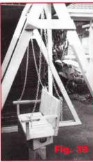
Connect four lengths of chain longer than required to the screw eyes with D shackles (**Fig. 38**). Keep some slack in the chain so the seat will drop about 50 mm when the boxes are removed (**Fig. 39**). Having excess chain is helpful as it allows you to adjust the seat height easily at this stage.
