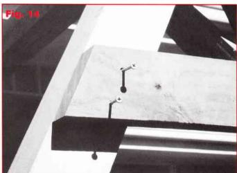
Add the angle braces (E), cutting the 45 degree angles on the workcentre. Drill and screw them to the cross rails with two 75 mm screws at each joint (Fig. 15).
