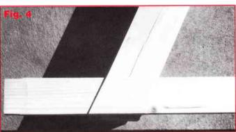
The frame sides have a housing cut out of them which forms the joint with the frame beam (B) cut later. Mark these housings in one set of frame sides. They are 25 mm deep in each frame side, and 90 mm long.
